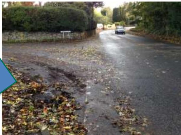
Figure 4: Lower drain on Driving Lane fleeced by mid-Autumn, cleared to indicate depth (2/11/14)
